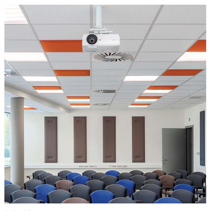
IN patented Snowsound® panels seamlessly integrate into standard 2' x 2' or 2' x 4' drop ceiling grids, either as a highlight or blending naturally with the existing colors. They offer superior acoustic comfort compared to traditional Acoustic Ceiling Tiles (ACT). This system is adaptable for retrofitting into existing spaces or specifying architecturally during the design phase. IN panels are compatible with the following grid systems: 15/16ths T-bar, 9/16ths T-bar, 9/16ths bolt slot.
