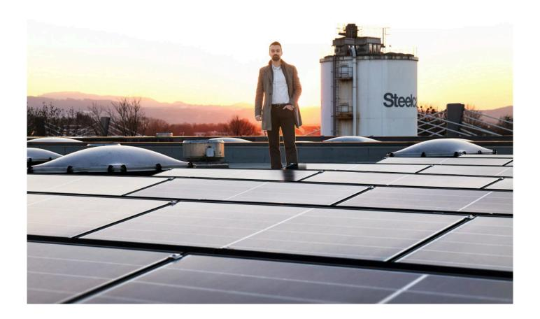
"The solar panels measuring 250 m<sup>2</sup> produce 30.000 kWh of electricity per year. When paired with the combined heat and power system, the Rosenheim Plant can produce about 50% of the plant's electricity requirements in the winter."
