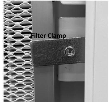
Repeat this process 3 or 4 times until the clamps are in a position nearly parallel to the face of the filter. **DO NOT OVER TIGHTEN THE CLAMPS.** If the clamps are over tightened the gel could be damaged and the filter seal may leak.
