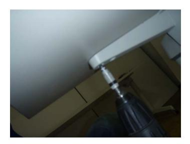
41. Fix the outer screws of the 4 cantilevers .
