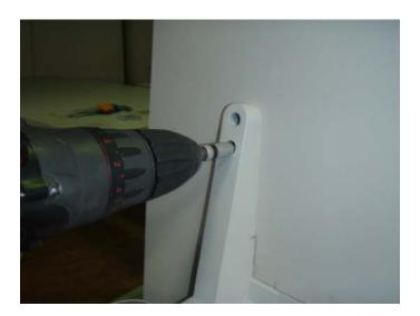
6. Loosen the inner screws of the 4 cantilevers.
