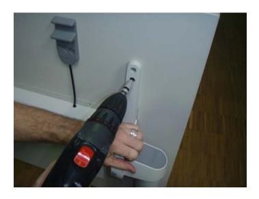
45. Fix the inner screws of the 4 cantilevers.
