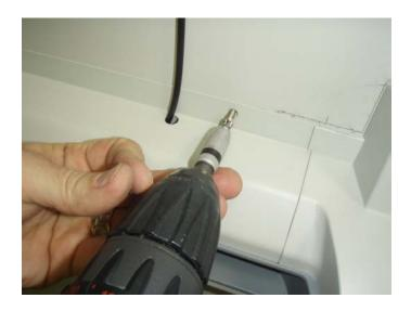
46. Tighten 8 screws of the cable tray.
