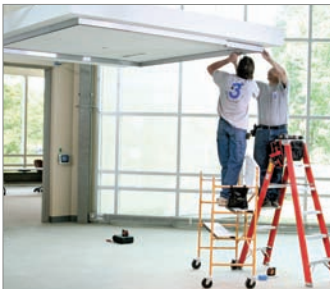
1. Install ceiling track
