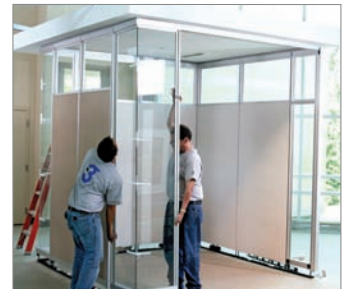
4. Install corner unit
