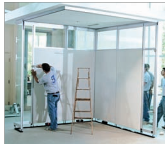
3. Connect wall panels with feature strips
