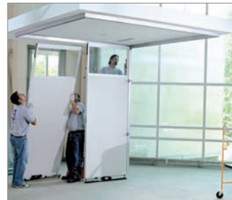
2. Insert wall panels into ceiling track
